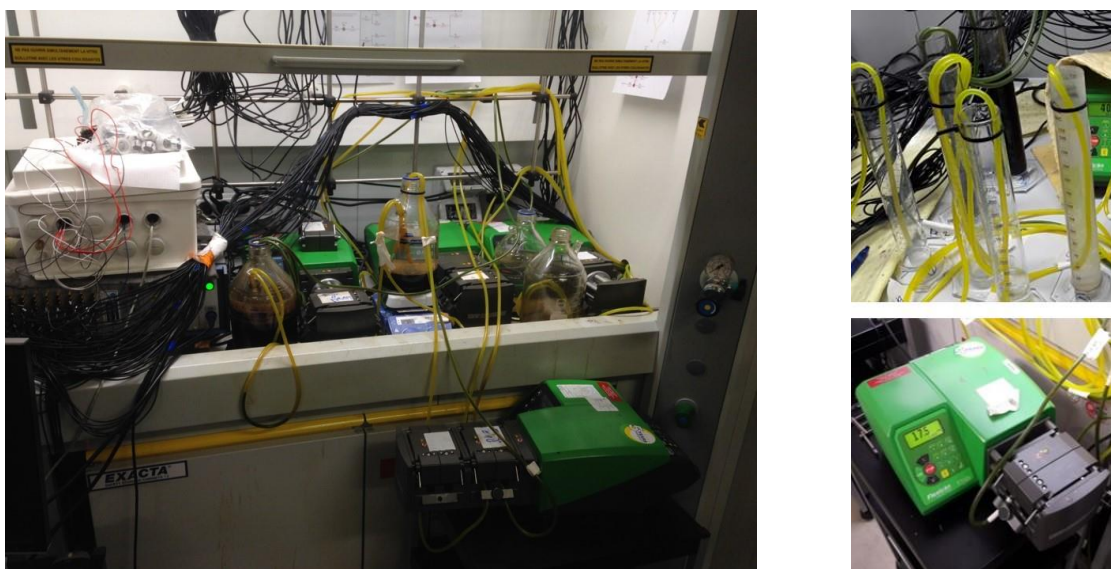
Figure 200: Photograph of the pumping and injection system for the 2D tank
