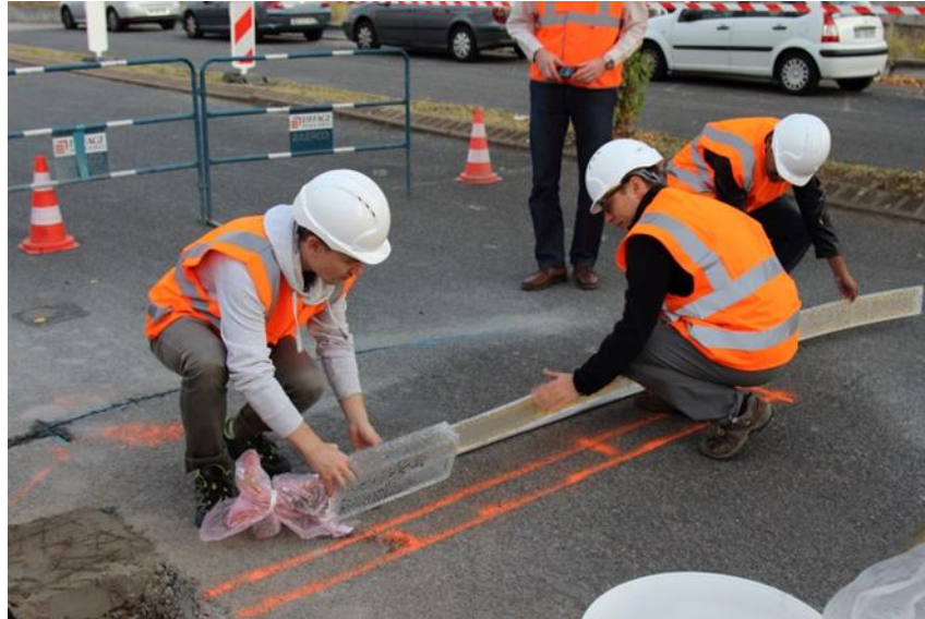
Figure 3.1 Altaroad's InTrack solution during installation on experimental construction site (October 2017).
