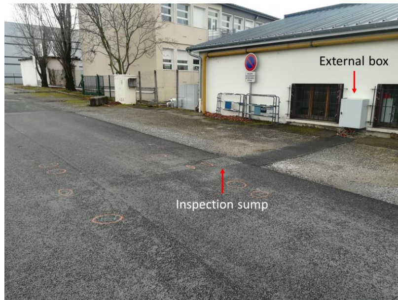
Figure 3.4 Experimental site: location of the external box and the inspection sump.
