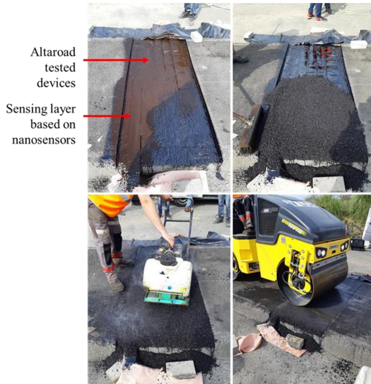
Figure 4.9 Different phases of the construction process: tack-coat emulsion application (top left), paving (top right), 1st compaction (bottom left), and 2nd compaction (bottom right).
