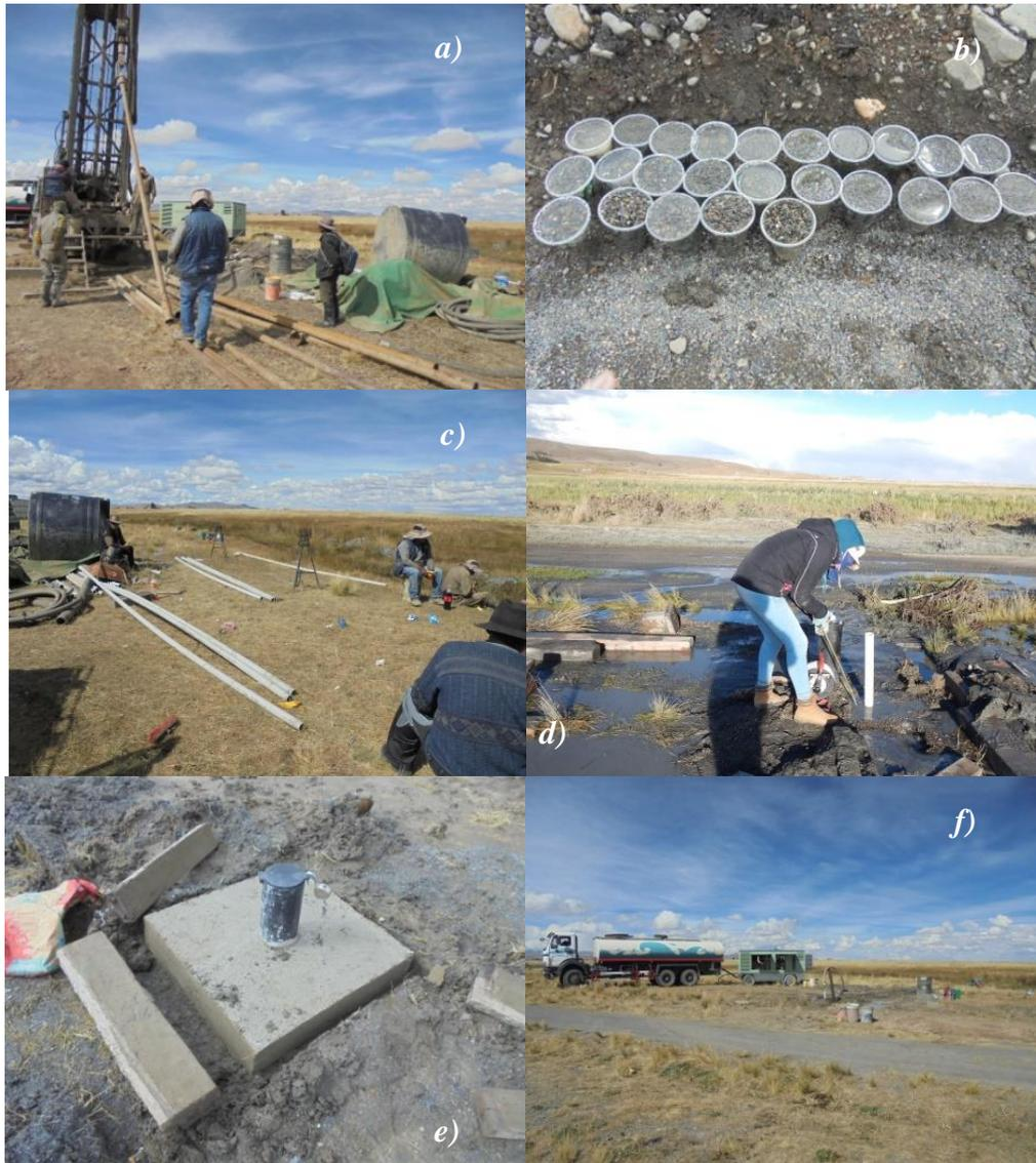
**Figure 3.8.** *Drilling and piezometer completion in the Katari and Lago Menor Basin. a) On-site drilling equipment, b) detailed stratigraphic record, c) PVC casing screening and installation of the piezometer, d) water level measurement after the development, f) Completion of the piezometer with a surface seal and a protective casing for providing piezometer security and e) piezometer development.*
