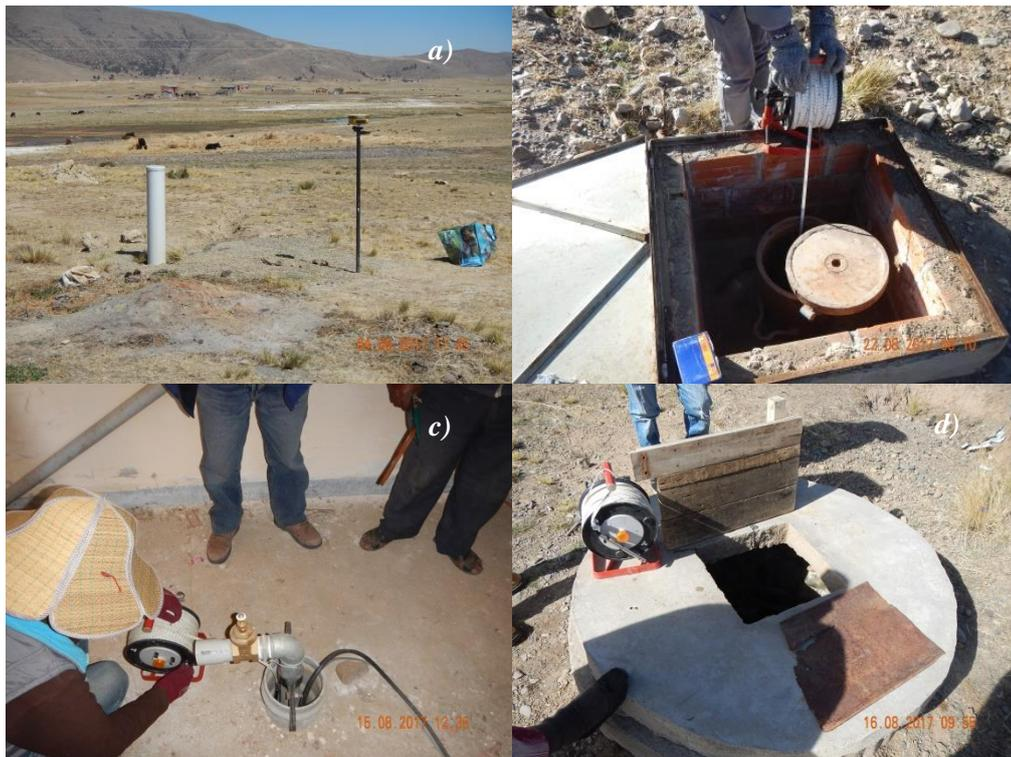
**Figure 3.5.** a) Device used for measuring the location of each inventoried groundwater source and example of groundwater level measurements performed in the field, b) deep well, c) well in a pumping house provided with a submersible pump and d) dug well.
