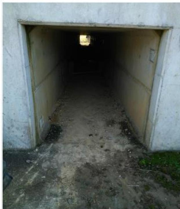
Fig. 1. Tunnel implemented under a railway as mitigation for the amphibian community (square concrete culvert 21 m length, 1 m high, 1 m width).
