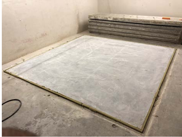
Figure 4.27: Emission room at Level Acoustics & Vibration.
