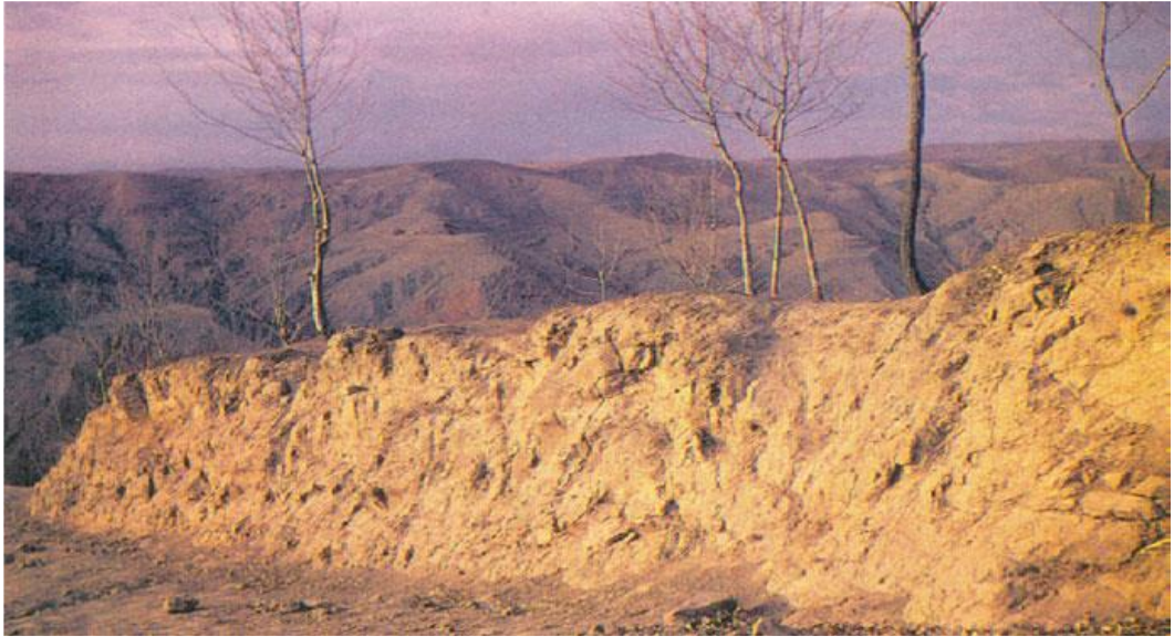
Figure 1.5: Section of the Great Wall of China built using the rammed earth technique around 2000 years ago (from Schroeder, 2016).
