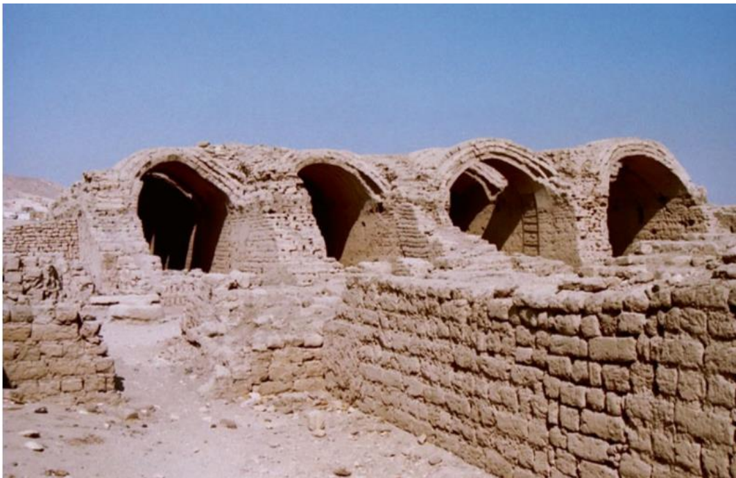
Figure 1.6: Earth block vault near Luxor/Egypt, around 1300 BC (from Schroeder, 2016).
