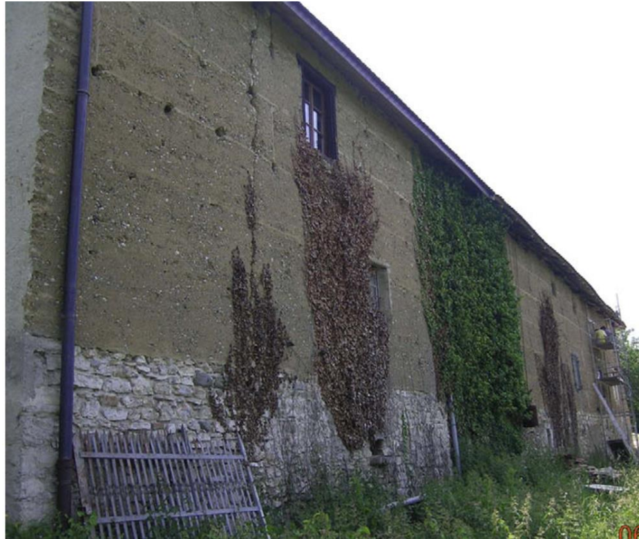
Figure 1.8: 150 years old rammed earth house in the South-East of France (from Bui et al., 2009).
