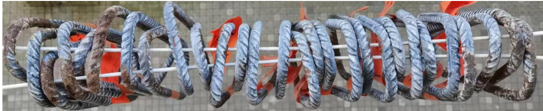
(a) Corrosion of horizontal legs in compressive zone
