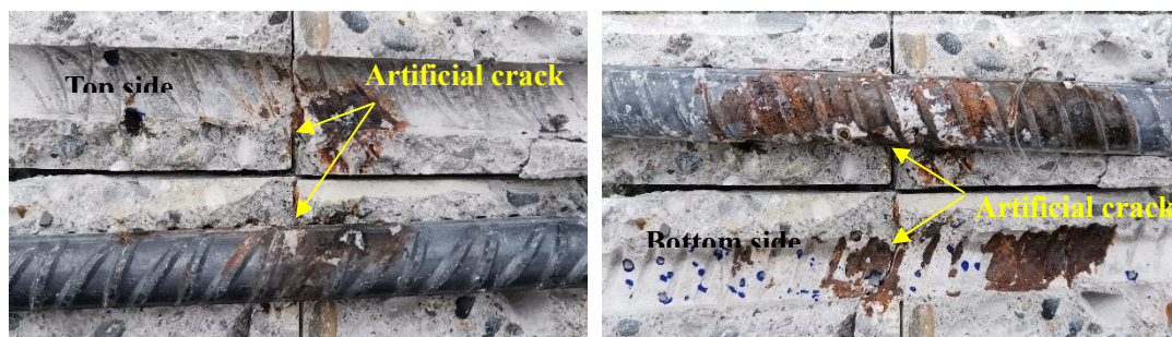
Figure IV-19. Corrosion pattern of top bar of B-1
