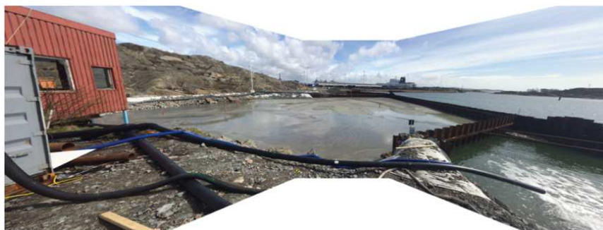
Cell 1 infilled with 50:50 GGBS:cement stabilised sediment
