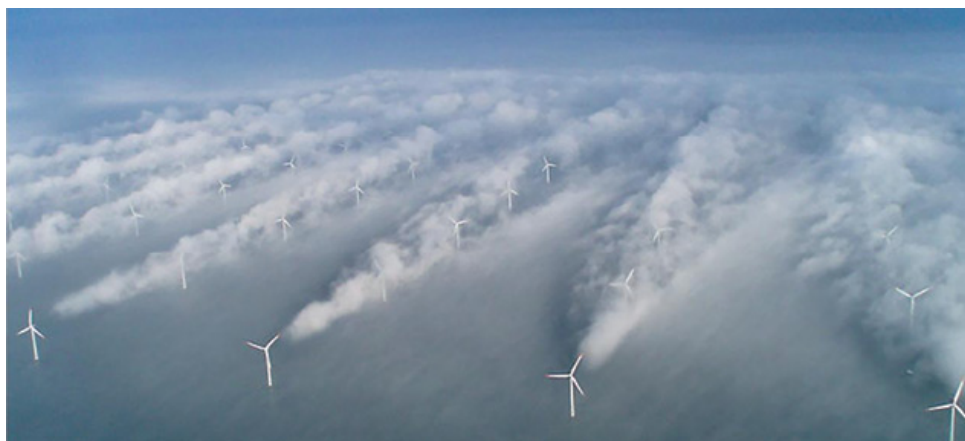
FIGURE 1.4 – Visualization of turbulence and eddies that a HAWT can endure. (Christian Steiness)
