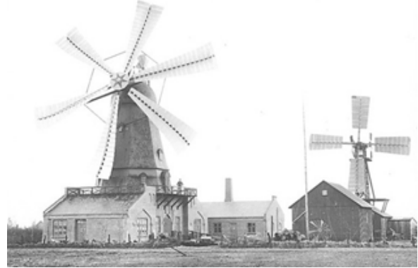
FIGURE 1.2 – First horizontal axis wind turbine in Askov, Denmark, photographed in 1897. ( www.windssofchange.dk )
