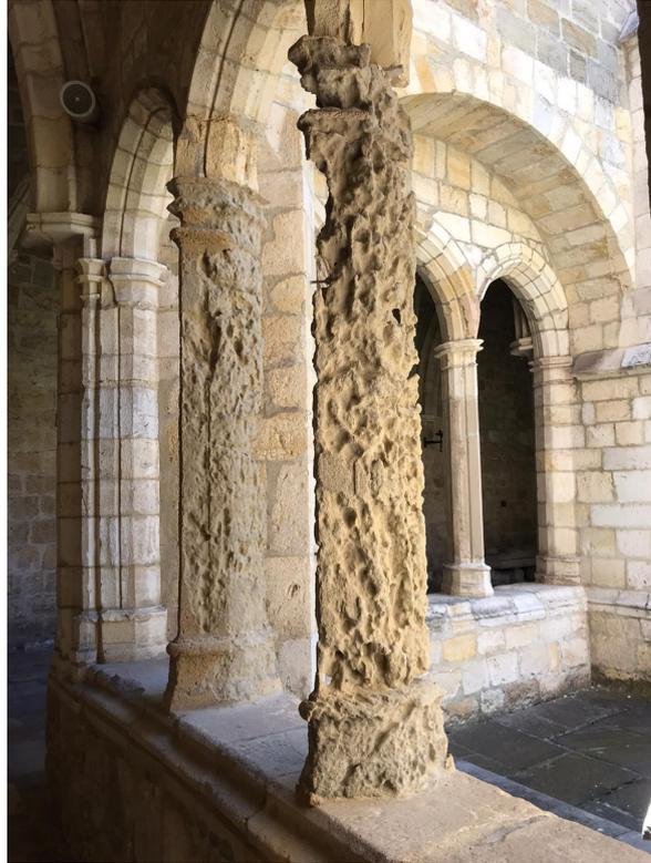
**Figure 1:** Detail of a pilar in the Santander Cathedral cloister weathered by salt crystallisation.
