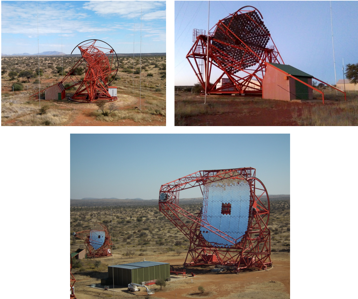
Figure 3.9: Different H.E.S.S. telescopes. Top: A close view of the 12-meter diameter H.E.S.S. telescopes (CT1-4) seen from different angles, showing the mechanical structure (left), and the segmented telescope mirror (right). Photographs taken during July 2018 shift on the H.E.S.S. site (A. Dmytriiev, 2018). Bottom: A close view of the large 28-meter H.E.S.S. telescope (CT5) (Credit: H.E.S.S. Collaboration, Frikkie van Greunen)
