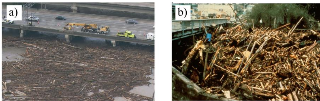
Figure I-1: Wood accumulations on the river channel, a) in Everett, USA, wood jam at the bridge on the Snohomish River (2019); b) In Soquel, USA, after January 1982 storm, logjam obstructed the bridge (Lassetre et al., 2012).
