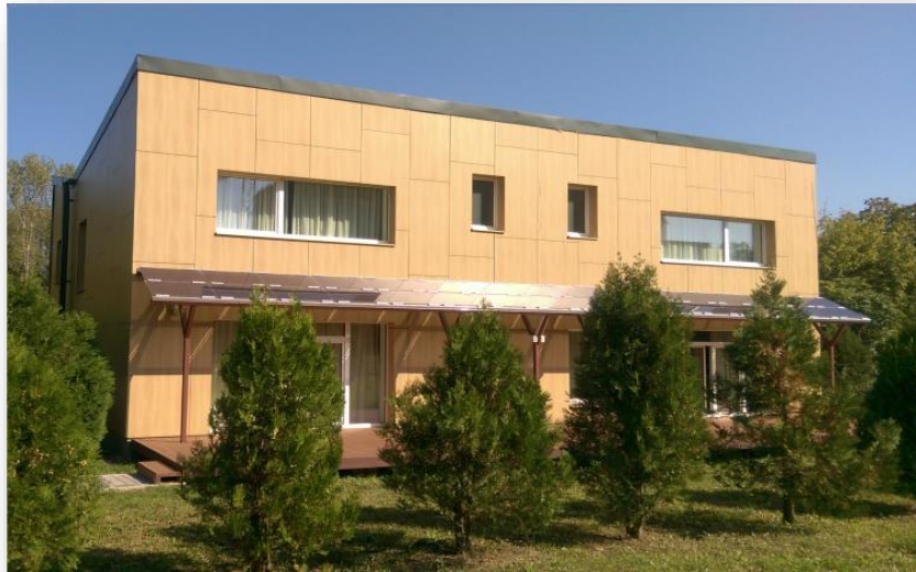
Fig. 2-1 UPB Passive House
