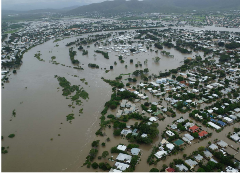
Figure 1.6: Flood of the Ross River in Townsville, Australia, on February 2019. Source of the photo: http://media.bom.gov.au/social/blog/2156/explainer-what-is-a-flood/ . Credit: Australian Defence Force.
