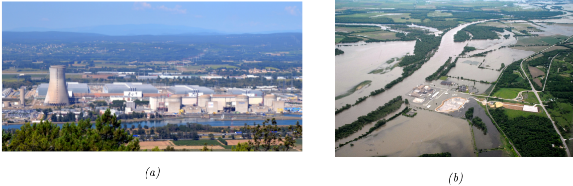
Figure 1.8: a) NPP of Tricastin, France (EDF). Source photo: https://en.wikipedia.org/wiki/Tricastin_Nuclear_Power_Plant . Credit: Marianne Casamance. b) Flood of Missouri River at the Calhoun NPP in Nebraska, 2011. Source photo: https://en.wikipedia.org/wiki/Fort_Calhoun_Nuclear_Generating_Station . Credit: U.S. Army Corps of Engineer.
