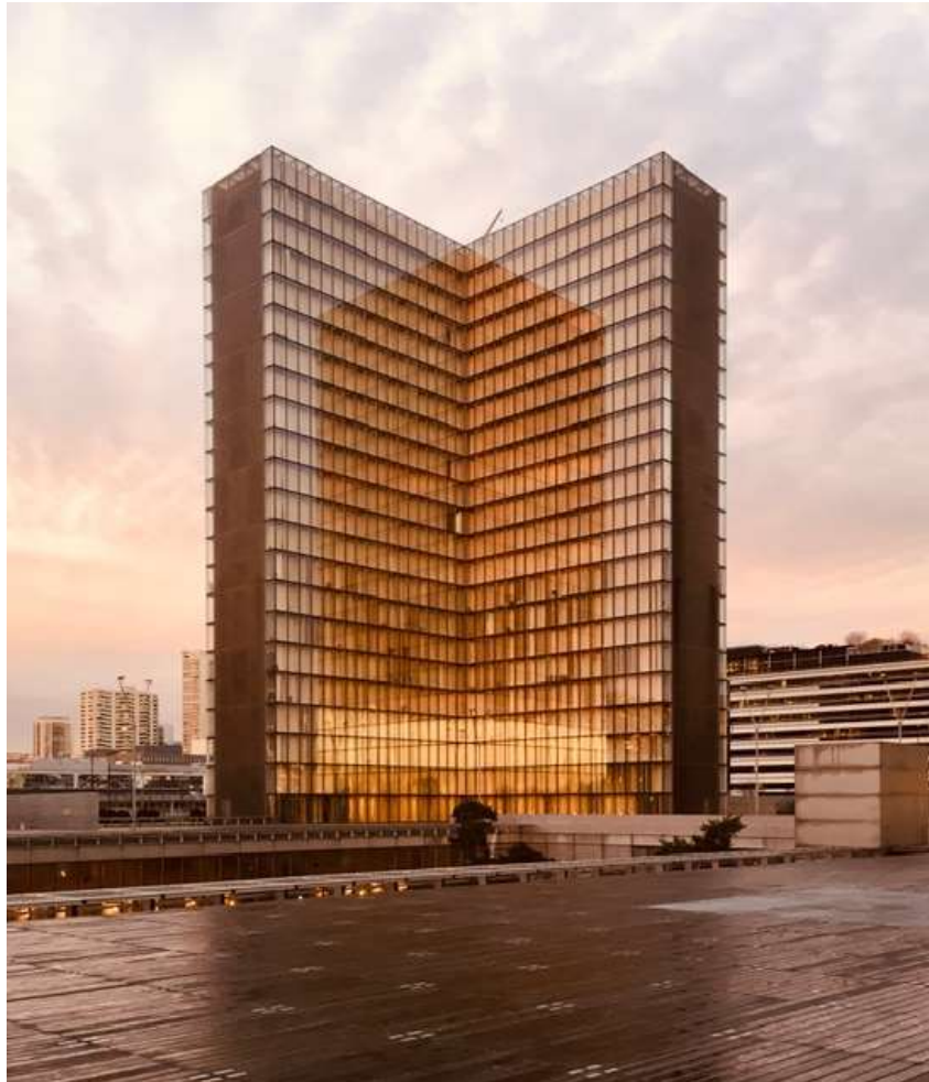
Figure 27 – Building forming a V, with windows generating several specular reflections between the two sides. Credits: Gaël Obein
