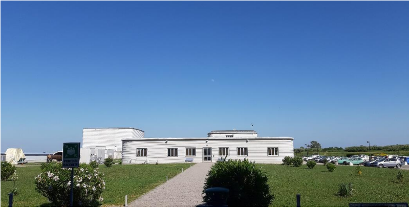
Fig. 4.6.1.a. Photo of the Control Room building. Source: Philippe Vincent
