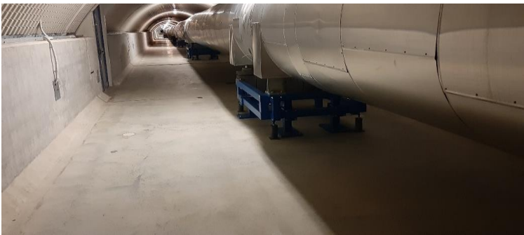
Fig. 4.6.1.n. The North gallery hosting the North 3 kilometers-long arm of the interferometer. Source: Philippe Vincent
