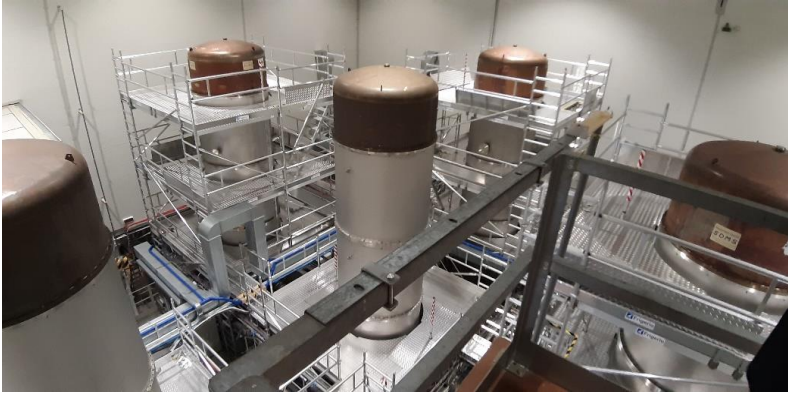
Fig. 4.6.1.j. Towers containing the superattenuators and the mirrors. Source: Philippe Vincent
