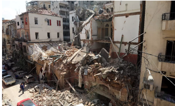
Figure 1.5 – A masonry building completely destroyed by the blast in Beirut (Lebanon). Photo credit: Mohamed Azakir, Reuters.
