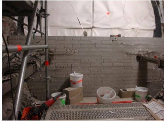
Figure 2-27 Construction of seal walls of bentonite/sand (40/60) bricks inside the drift for the NSC experiment (de la Vaissière et al. 2014).
