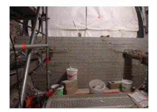
Figure 2-27 Construction of seal walls of bentonite/sand (40/60) bricks inside the drift for the NSC experiment (de la Vaissière et al. 2014).
