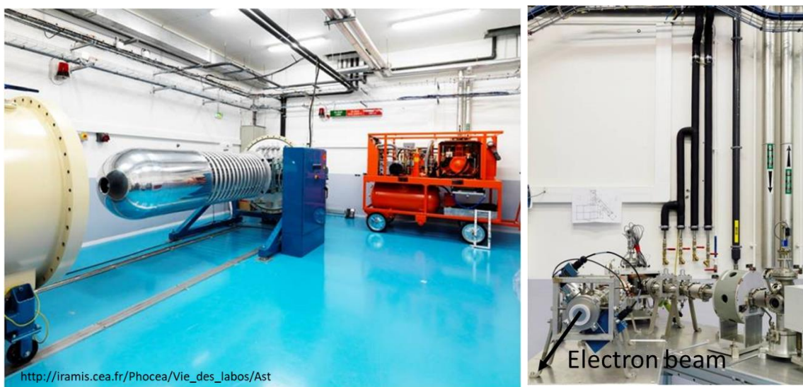
Fig. II-26 View of SIRIUS platform facility, left: accelerator tank, right: irradiation beamline.
