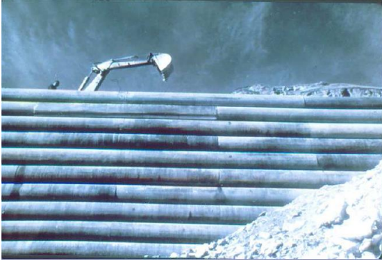
Figure 1-2 First reinforced soil retaining wall constructed in 1965 by EDF (Chéret, 2015)
