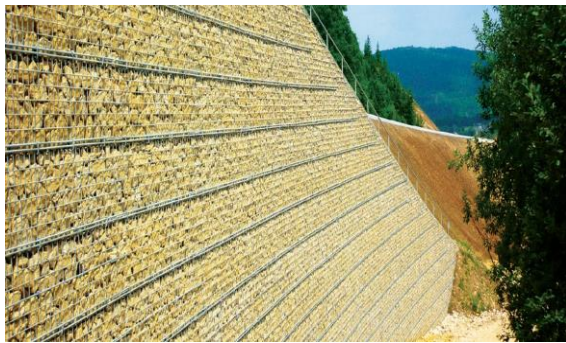
(c) Gabion facing
