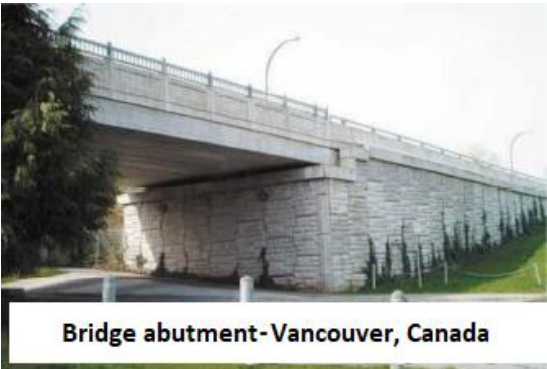
(c) Bridge abutment
