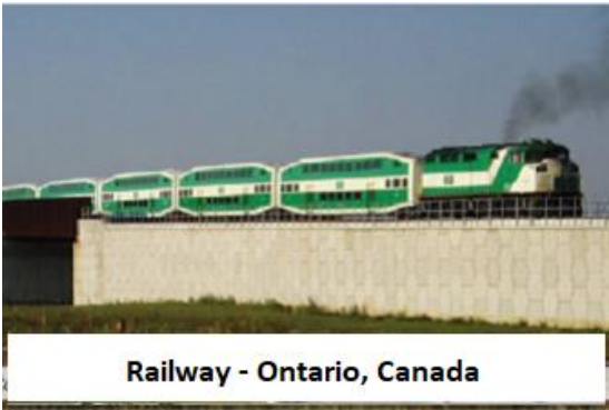
(b) Railway structure
