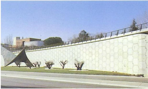
(a) Precast concrete panels
