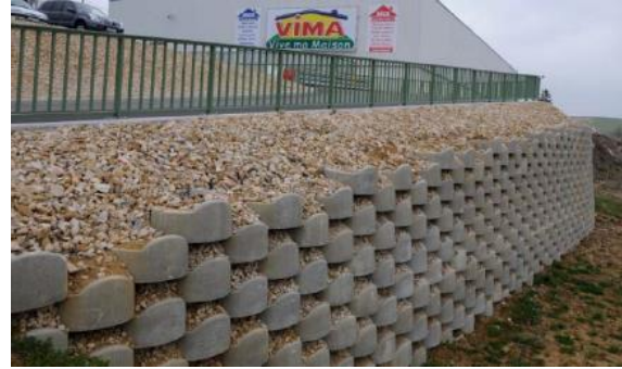
(b) Dry cast modular block wall units
