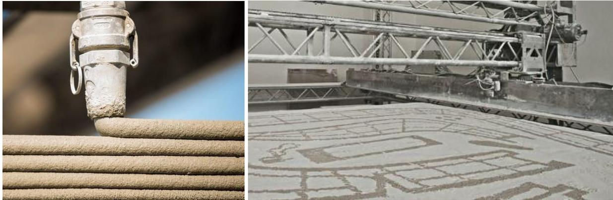
*Figure 8: Difference Between (Left) Extrusion-Based [38] and (Right) D-Shape [39] AM approaches*
