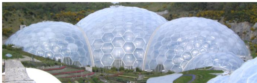
Figure 4.22: The hexagonal gridshell of the Eden Project in Cornwall, England (picture in public domain)
