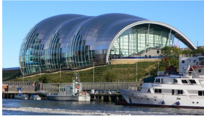
Figure 3.15: The SAGE Music Centre in Gateshead is a moulding surface, a particular class of surfaces with planar curvature lines (© Jim F. Bleak)
