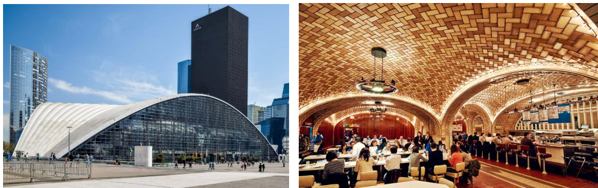
Figure 1.2: Left: The concrete shell of the CNIT (©Alexandre Prevot). Right: Guastavino vault of the Grand Central Oyster bar in Manhattan (©Flicker4Jazz)
