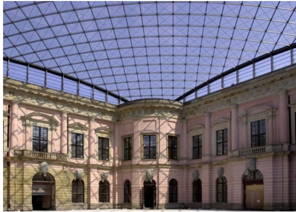
Figure 2.19: The roof of the German History Museum is a translation surface (©Kai-Uwe Heinrich)
