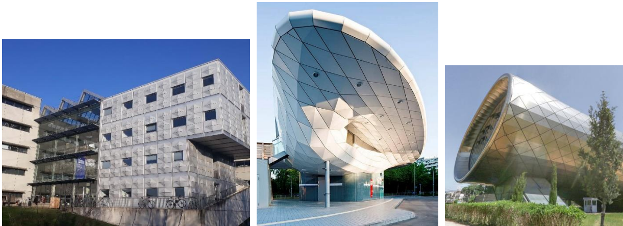
Figure 4.9: Diagonal folds on facades. Left: EAVT in Marne-la-Vallée (Picture: X. Tellier). Middle: Hamburg Poppenbüttel Bus Terminal (© www.archimages.de). Right: Rhike Park Music Theater (© Aslan Juan)
