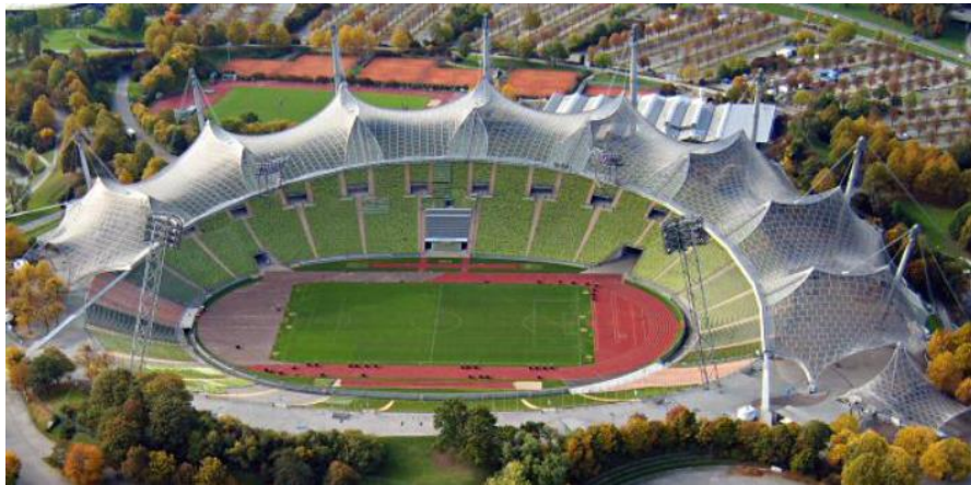
Figure 5.4: The geometry of the cable net of the Olympic stadium at München is based on a minimal surface (picture in public domain)
