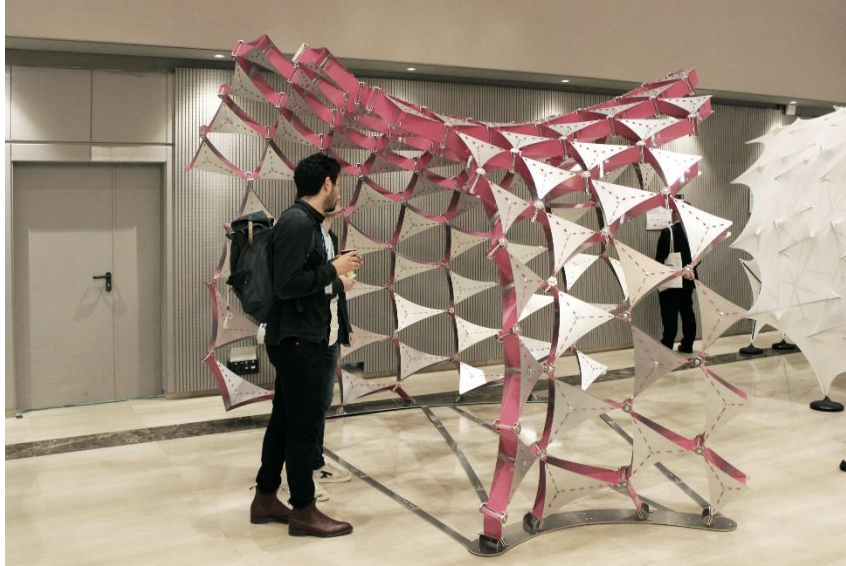
Figure 4.2: The Caravel heX-Mesh pavilion at the IASS 2019. The geometrical properties of Caravel meshes are used to simplify and standardize all the connections.
