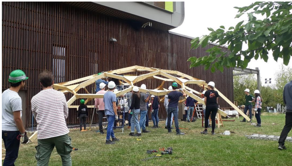
Figure 4.40: Erection of the pavilion Construire le Courbe 2019
