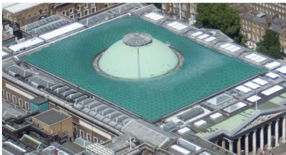
Canopy of the great court of the British Museum. The steel gridshell follows a triangular mesh.
