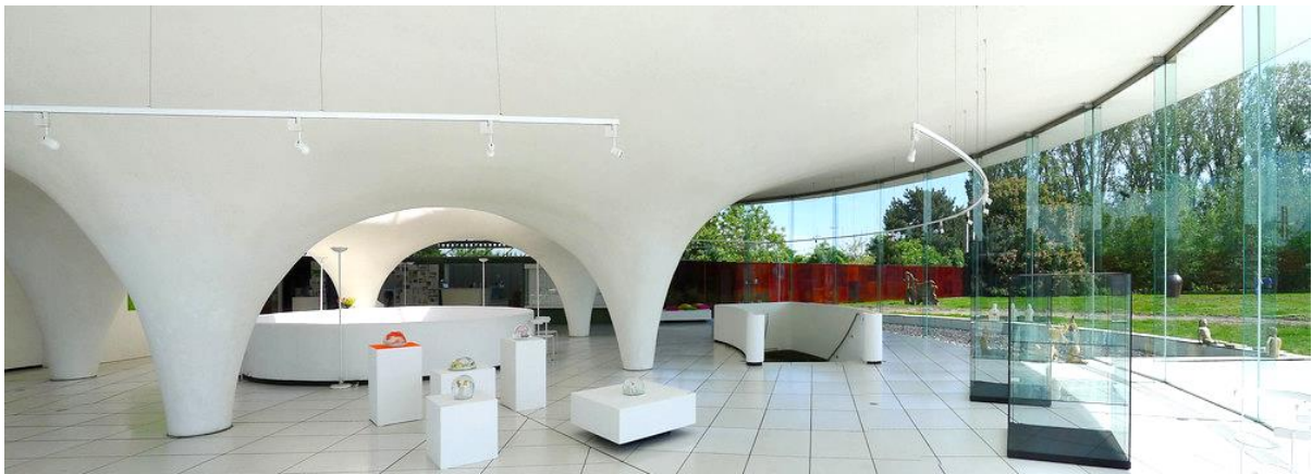
Figure 6.34: The concrete shell of the Keramion museum in Frechen, Germany, is a Pelikan surface – a special type of i -LW surface also referred to as i -minimal. ©Klaas Vermaas
