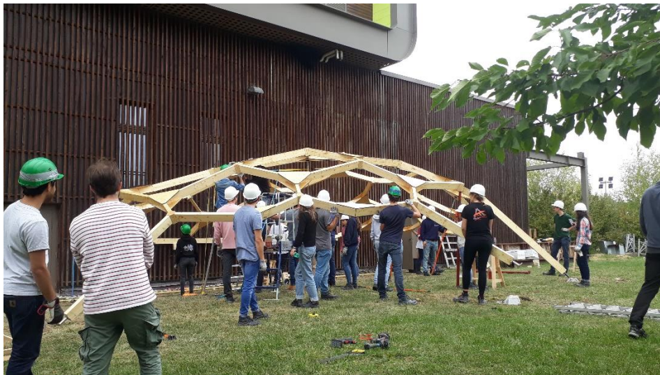
Figure 4.40: Erection of the pavilion Construire le Courbe 2019
