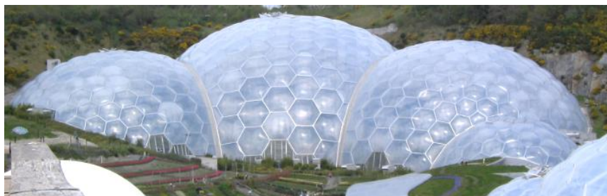
Figure 4.22: The hexagonal gridshell of the Eden Project in Cornwall, England (picture in public domain)
