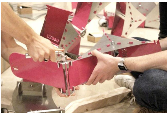
Figure 4.39: Details of the Caravel heX-mesh pavilion. The pavilions is made of planar laser-cut sheets, bolts, and standard stamped 120^\circ connectors.
