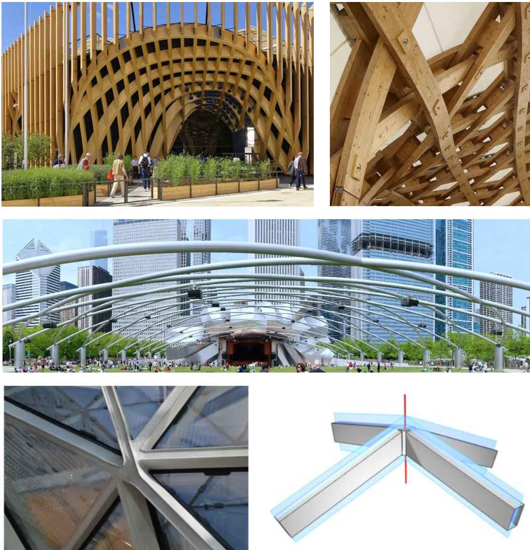
Figure 2.4: Common strategies to deal with geometrical torsion: i/ Set all the beams in vertical planes (Top left - Picture courtesy of Simonin) ii/ Twist beams (Top right - ©Didier Boy de la Tour) iii/ Use circular profiles (Middle - picture in public domain) iv/ Accommodate torsion at nodes (Bottom left - ©Romain Mesnil) v/ Find a torsion-free beam layout – Example of a torsion free nodes (Bottom right)
