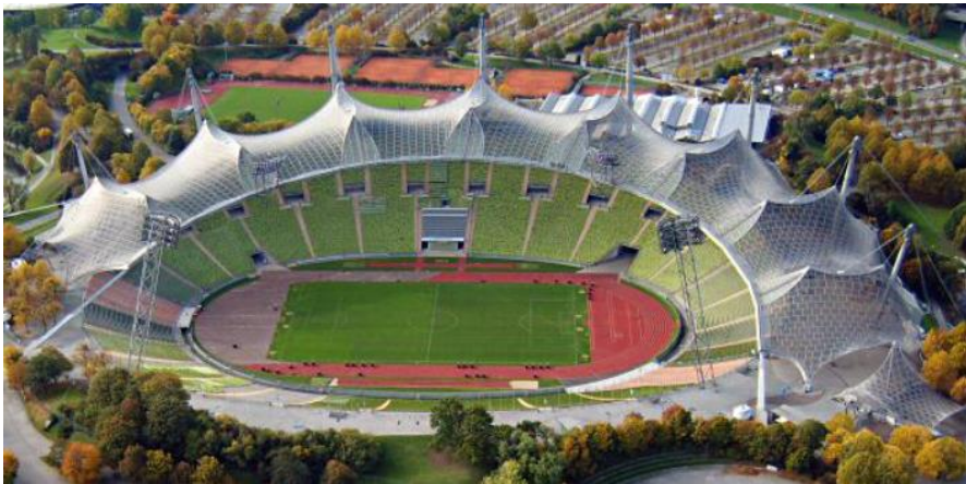
Figure 5.4: The geometry of the cable net of the Olympic stadium at München is based on a minimal surface (picture in public domain)
