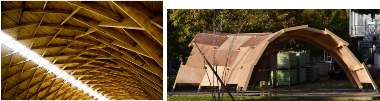
Figure 2.5: In a nexorade, beams are connected two by two. Left: Lamella roof at Auburn University's Rural Studio (©James Diewald) Right: Hybrid shell-nexorade, Navier laboratory.
