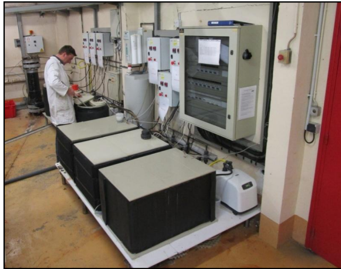
Figure 19 : Sea water aging tanks at Ifremer
