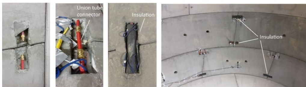
Figure 4.8: Pipes connections between adjacent segments.
