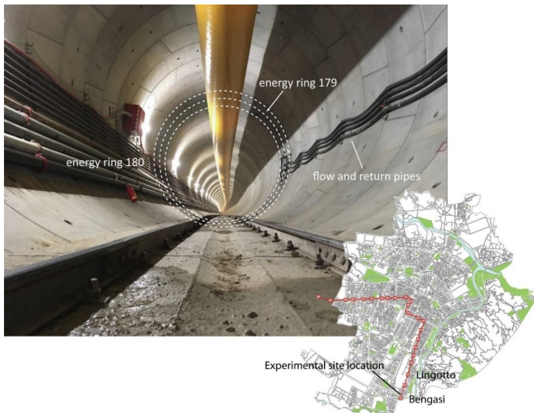
Figure 4.1: View of the Enertun experimental site and its location along the Turin Metro Line 1.
