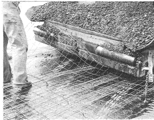
Figure 2-24. Installation of steel mesh for reinforcement of pavements in Michigan/USA (Williams 1953)
