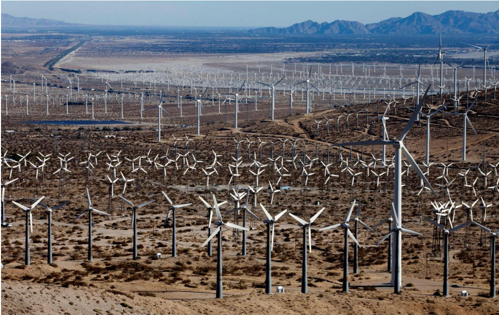
FIGURE 9: San Geronio Pass wind farm [5].
