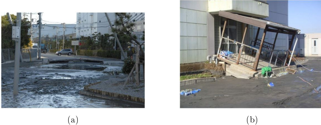
Figure 2.3: Destruction of the ground due to liquefaction in the Tokyo Bay area: spreading of sand over the road (a); Offset between an undamaged building and settlement of the surrounding ground (b) (Ishihara et al., 2011)
