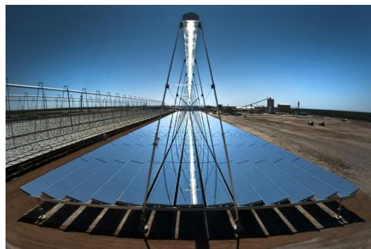
*FIGURE I-15 Areva Solar's Linear Fresnel Reflector, Bakersfield, CA, USA [76].*
