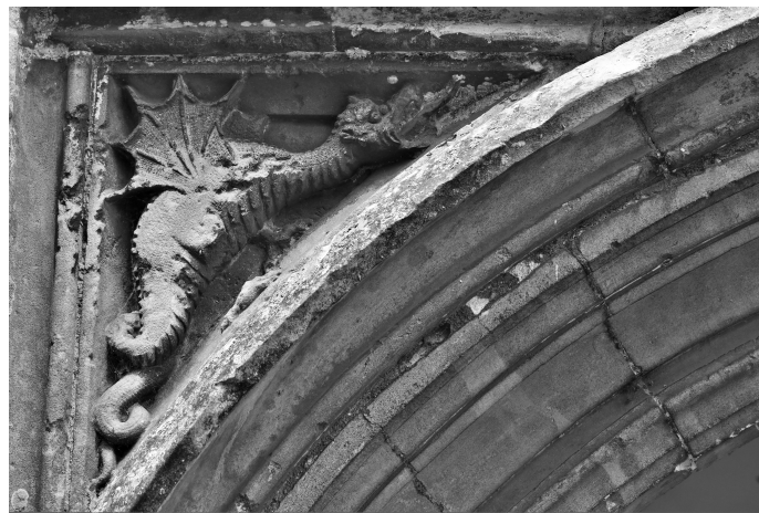
Figure 3.1: Example of an architectural spandrel in the doorway of the Saint Georges Church in Great Bromley (Essex, UK). The spandrel is decorated with a Dragon, as part of the representation of Saint Geroge’s legend. Picture adapted from an original photography by Michael Garlick (CC BY-SA 2.0)
