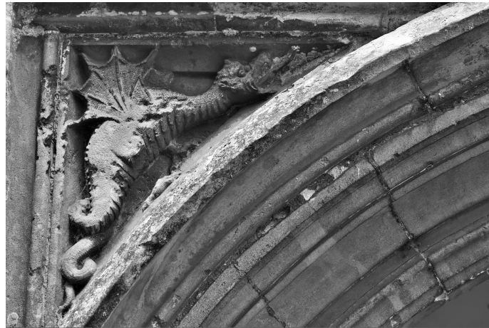
Figure 3.1: Example of an architectural spandrel in the doorway of the Saint Georges Church in Great Bromley (Essex, UK). The spandrel is decorated with a Dragon, as part of the representation of Saint George's legend. Picture adapted from an original photography by Michael Garlick (CC BY-SA 2.0)
