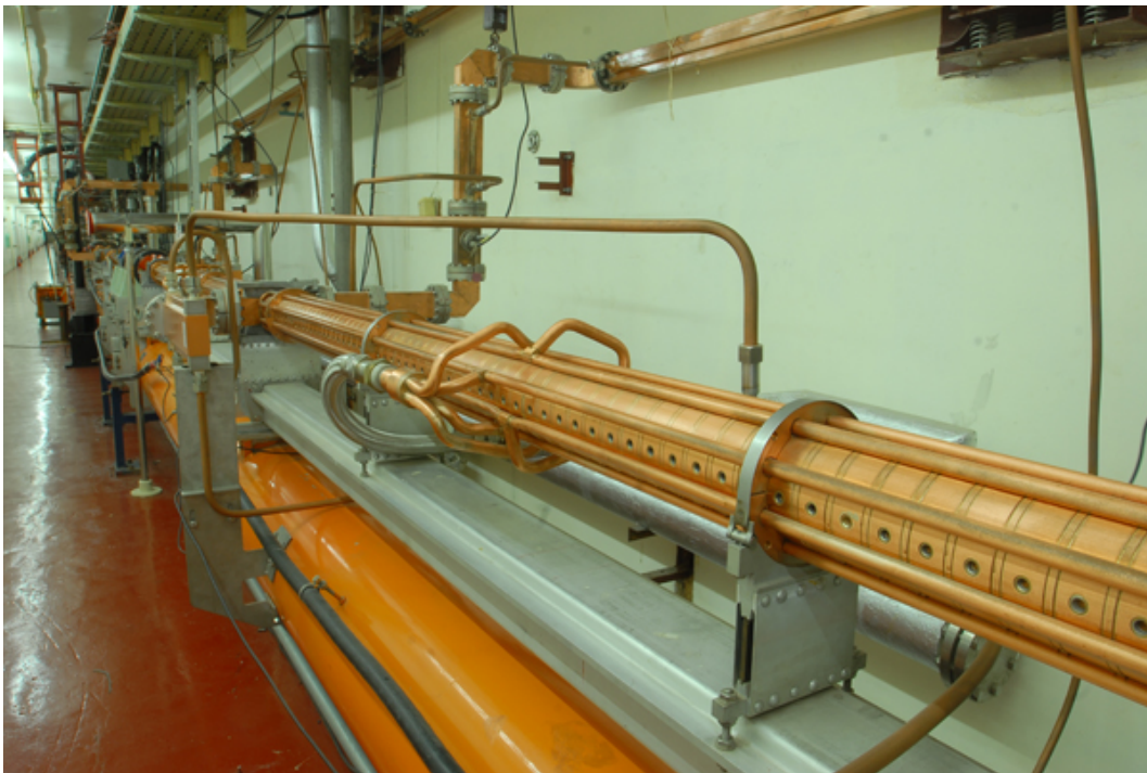
Fig. 2.16 Normal conducting S-band periodic accelerating structures in BEPCII [73]
