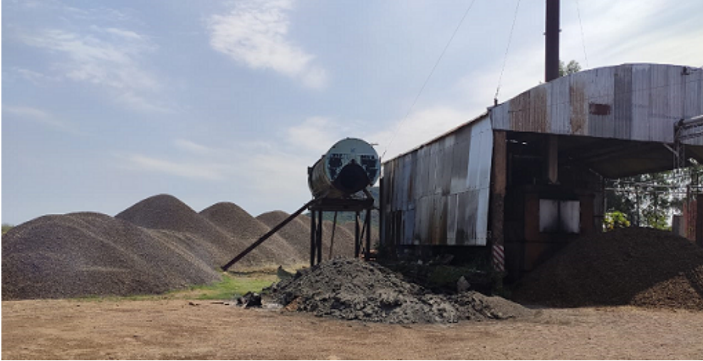
Figure 1.13: Coconut endocarp to be used in boilers. Courtesy of OISA S.A.
