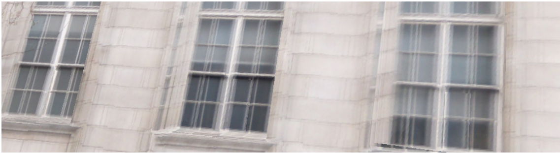
Figure 3.13 – Misalignments introduce ghosting when performing image-based rendering using the original images and the refined mesh.
