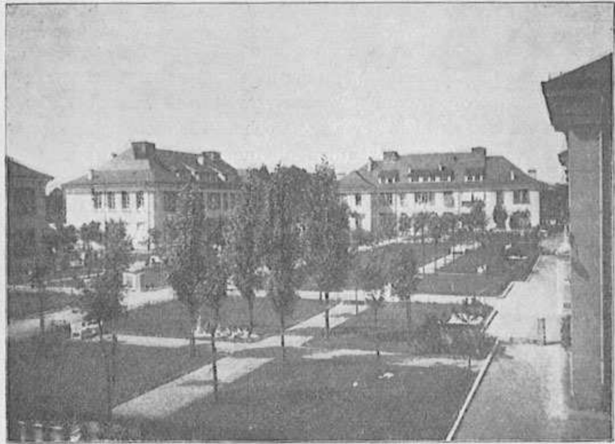
Figure 2.1.: Image of the the Kinderklinik from Adalbery Czerny (1911), illustrating the pavilion structure. 134
