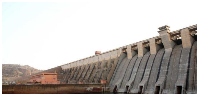
Figure 28 barrage de Manantali, source OMVS.
