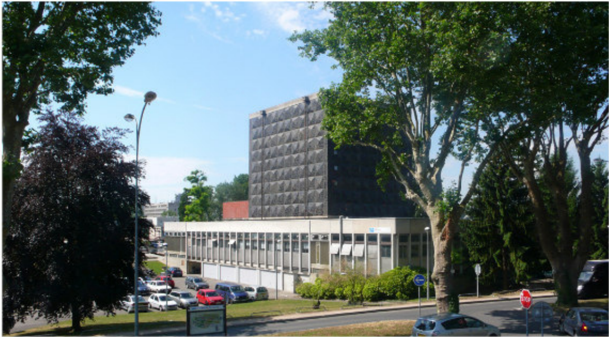
Figure 2.1: Photo of the IP2I Haefely building. The cryogenic facility is located in the basement, at the same height as the parking lot.
