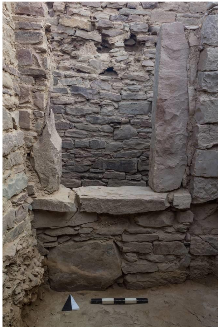
Figure 50: Entrance of Building F-b1 East flanked by two vertical stones (SU 3973 and SU 3966) and the threshold (SU 8686), view from R17 in the interior to the exterior. Wall SU 3969 can be seen in the background (Building F-b3 roofing, see Figure 25); view from S (© DAI Orient Department 2016 F. Weigel)
