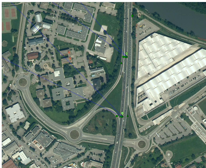
Figure B.2: Aerial photo of intersection 1. Location of the magnetic loops are shown with dark-green dots. The off-ramp is labeled with a light green marker with an "O".
