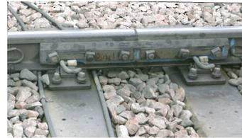
Figure 2.5: Rail Joints and the fastening on sleepers [169]
