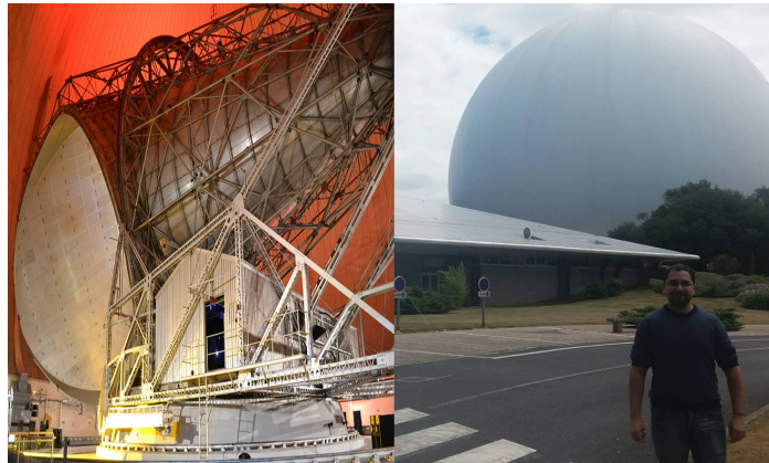
Figure 4.1 – Pleumeur-Bodou Ground Station For Satellite Broadcasting [71]
