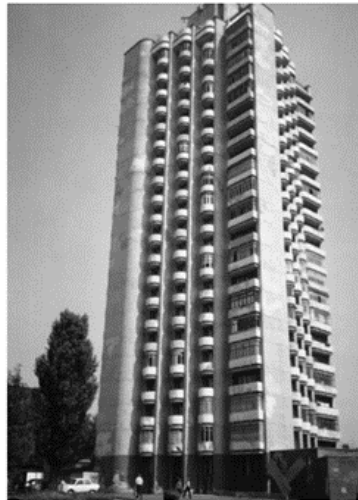
Figure 1.9: A 24-storey building built with alkali-activated slag cement concrete on Berezinsa street 2, city of Lipetsk, Russia, 1994 (Shi. et al., 2006)
