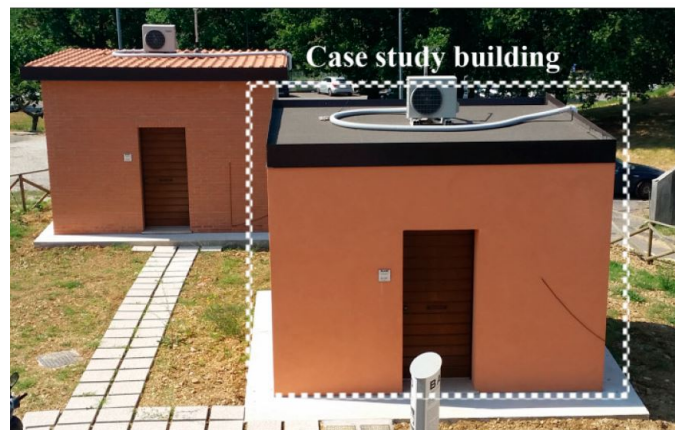
Figure 2.12.: Picture of the test-room facility used in Bianchi et al. [20].
