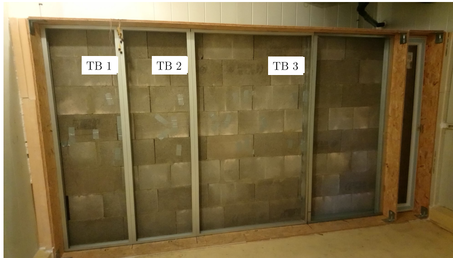
Figure 4.13.: CEREMA: Wall before installation of the glass wool and gypsum boards.
