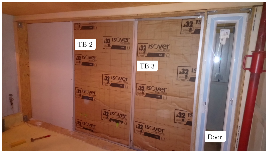
Figure 4.14.: CEREMA: Wall before the installation of the gypsum boards.
